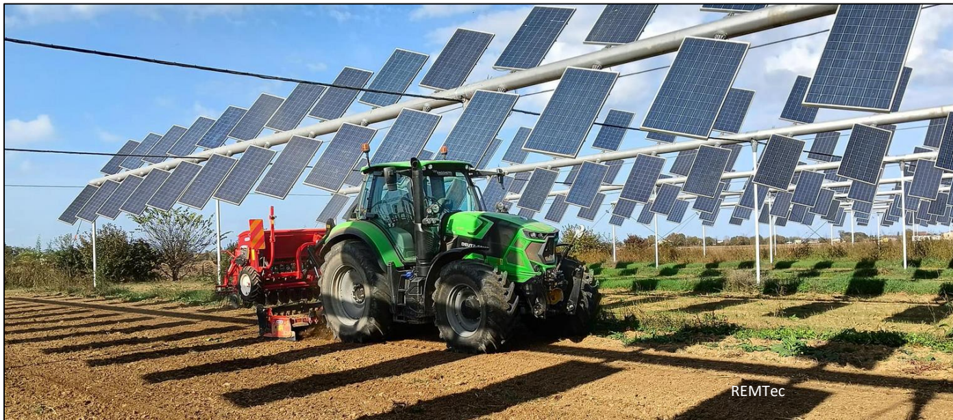
Illustration of the planned Agri-PV research facility at the ZHAW campus with dynamic dual-axis orientation of the modules
