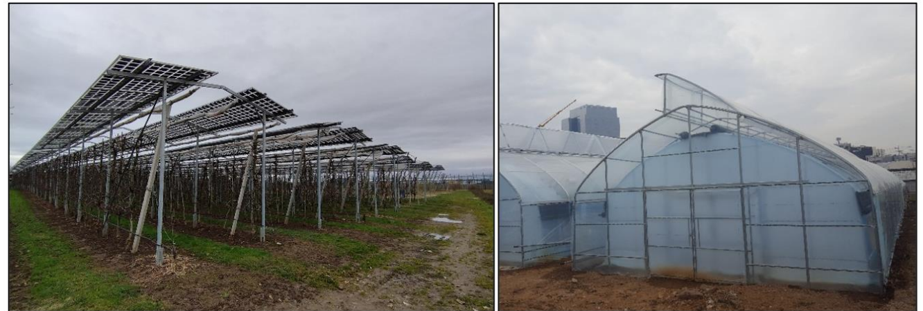
Figure 2. Left: Overhead agrivoltaic system with open sides, generating partial shade and solar electricity. Right: Greenhouse with semi-cylindrical roof and closed sides, with vents for climate control, adapted from (Akpenpuun et al., 2021).
