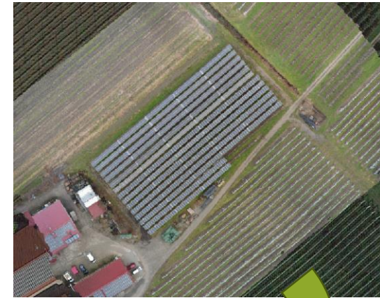
Current installation of solar panels
